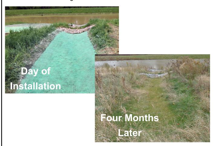
Recyclex TRM protected the seed and soil while creating optimal growing conditions to provide long-term vegetation reinforcement to this channel. Recyclex TRMs have a light color that prevents seed burn-out. Approximately 18 plastic bottles are diverted from landfills for every pound of Recyclex fibers. Recyclex fibers don't float, which ensures your soil is covered during hydraulic events..
