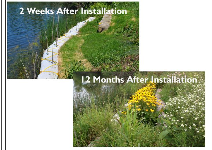
Curlex Blocs are a versatile solution suitable for shoreline restoration applications with low energy wave action. In this installation Curlex Blocs were used with live Willow cuttings, native sod, native seeding and Curlex erosion control blankets to restore and protect this site.
