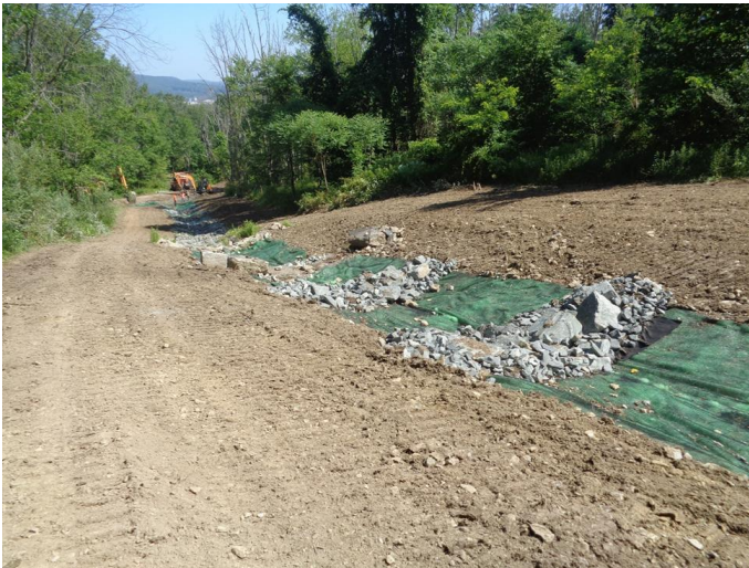
Figure 8. TriNet Recyclex and New Rock Check Dams
