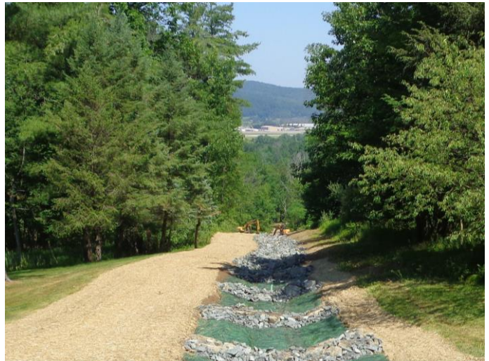
Figure 9. AEC Premier Straw Installed Outside Channel
