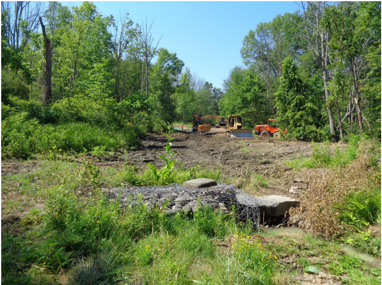
Figure 5. Removal of Existing Rock and Channel Reshaping
