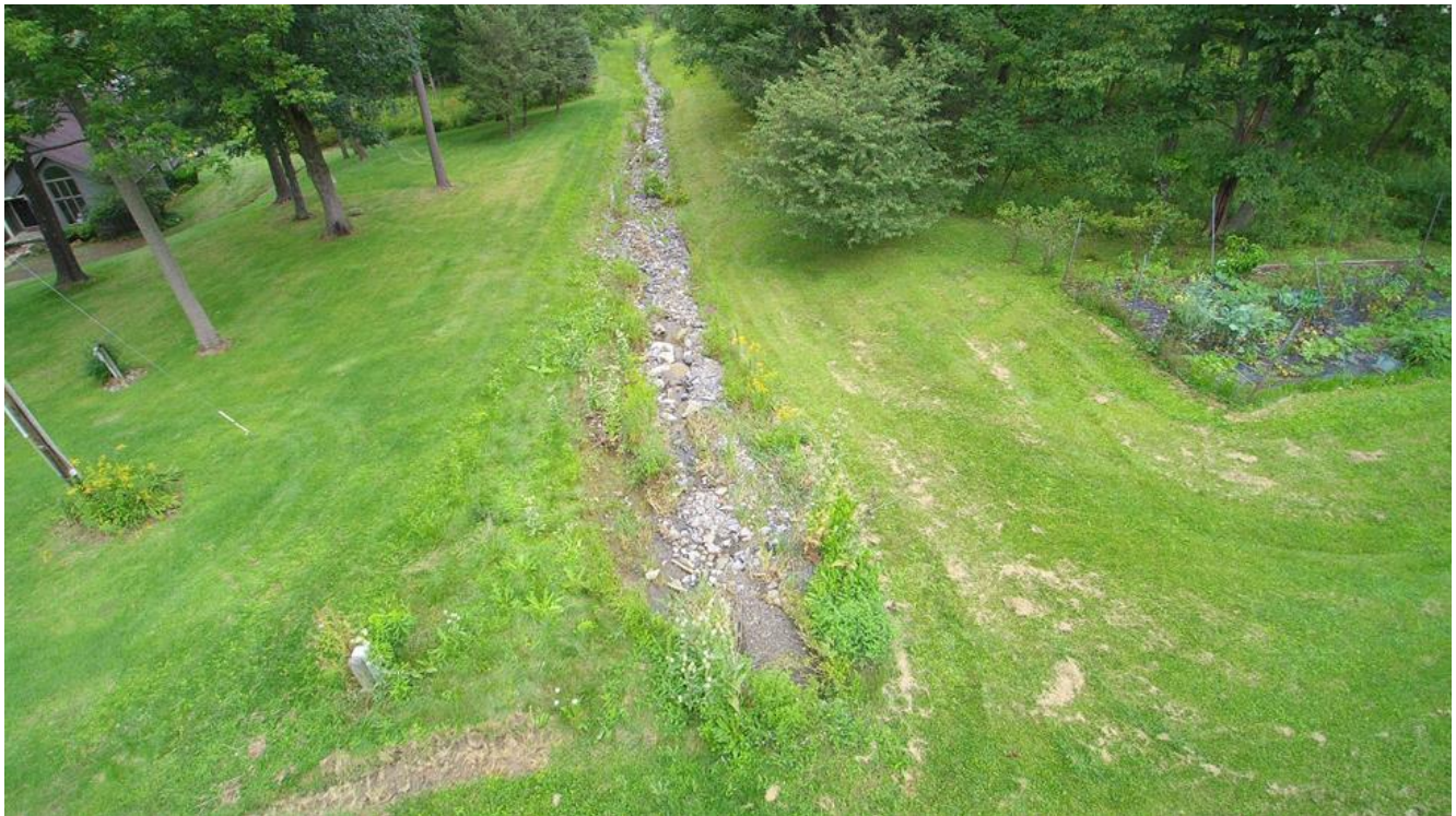
Figure 2. Outdated and Eroded Stormwater Channel
