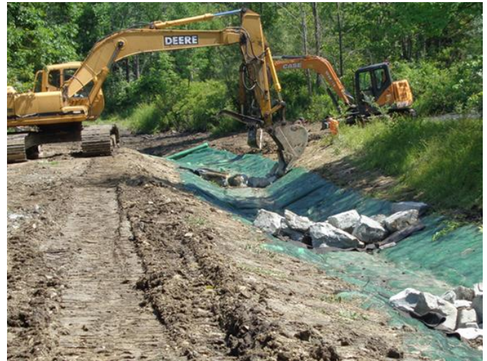
Figure 7. New Rock Check Dams Over TriNet Recyclex
