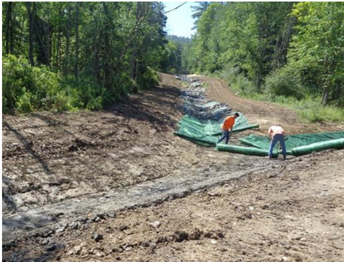
Figure 6. Installation of TriNet Recyclex
