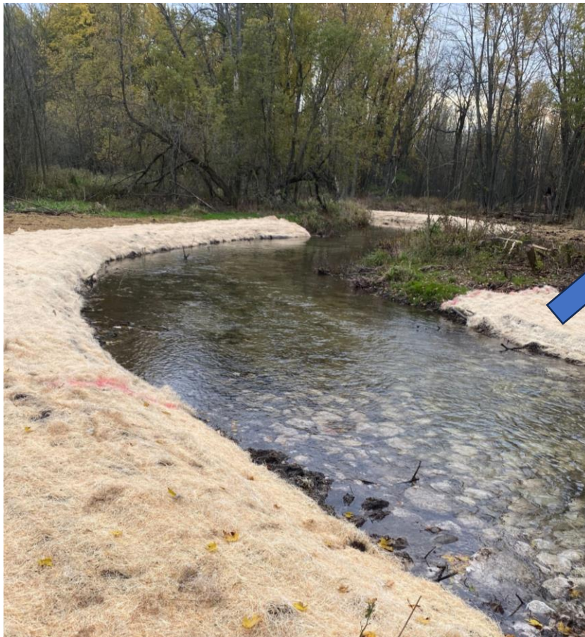
Figure 7: Curlex NetFree, a naturally seed-free erosion control blanket, protecting the precious trout stream after rip rap was added to improve flow conditions and before native seed mix germinated.
