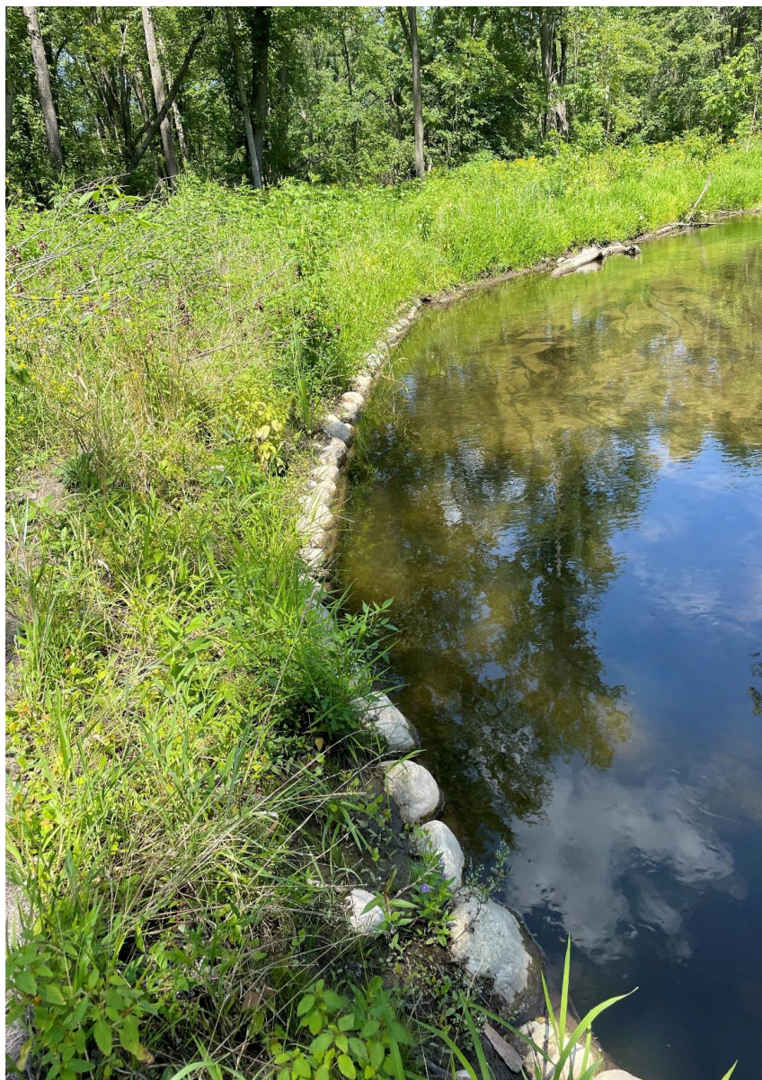
Figure 6: Vegetation on lunker structure under bank from Figures 4 & 5 that was protected with Curlex NetFree erosion control blanket approximately one season after installation.
