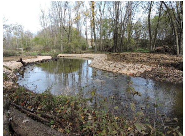
Figure 11: "During" photo of Curlex NetFree protecting restored bank section shown in Figure 10 shortly after installation.
