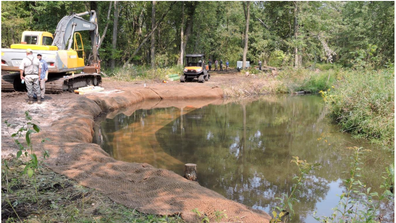
Figure 4: Completion of lunger structure before final backfilling, seeding, and covering. Note black locust post near center of photo that had not been cut off yet.
