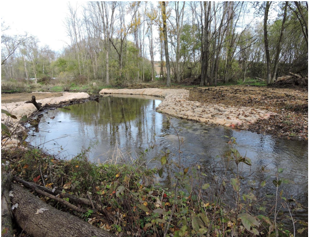
Figure 5: Completed lunger structure from Figure 4 protected with Curlex NetFree erosion control blanket.
