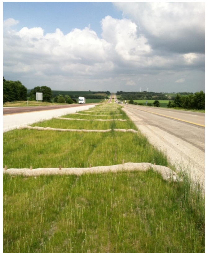
Figure 6. After (July Year One): The challenging highway median is becoming permanently stabilized by vegetation only approximately two months after installation of Curlex® II .98 erosion control blankets and Curlex® Sediment Logs.
