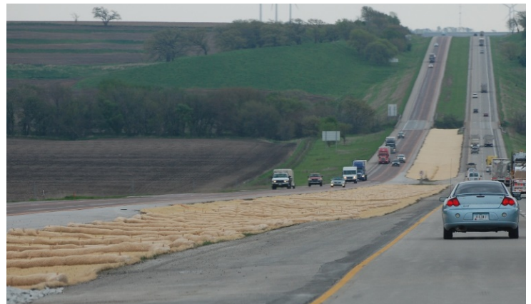
Figure 5. (May Year One): Curlex® II .98 erosion control blankets are double-netted for higher performance. They were installed in conjunction with Curlex® Sediment Logs which are porous and engineered to both dissipate velocity and filter stormwater runoff before the median discharges into the Nishnabotna River. Both products are made from sustainably harvested Great Lakes Aspen excelsior fibers.
