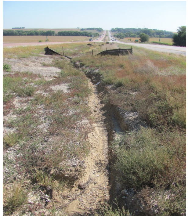
Figure 4. Scour under damming device caused severe erosion. These failures led to complete rework of the area with Curlex® II .98 erosion control blankets and Curlex® Sediment Logs.
