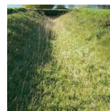
Vegetated Recyclex® TRM channel.
