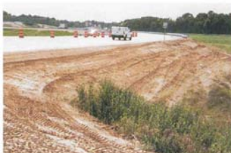
Prior to installing CurlexGRASS, the shoulder subgrade is properly prepared and seeded.
