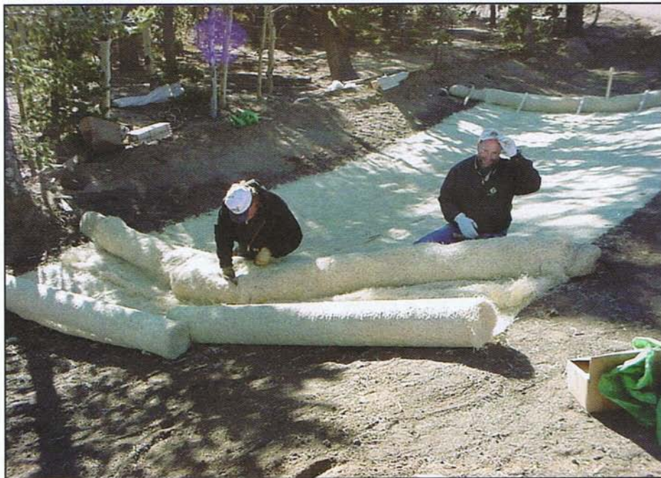
Temporary erosion control blanket (ECB) over the soil loaded TRM.
