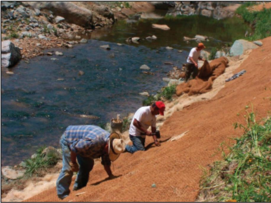
**Installation of coir woven mat on top of net free excelsior using one foot long wood stakes. Photo taken May 2005 by Pete Romocki.**
