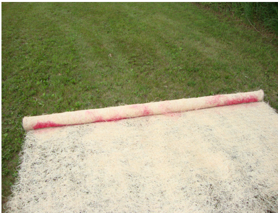
Figure 1. Locate red dye line near the end of the RECP.
