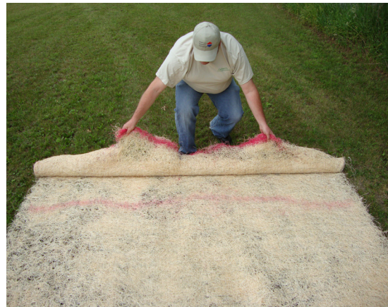
Figure 2. Pull end of RECP along red dye line.
