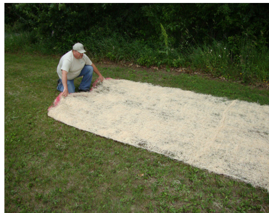
Figure 4. Properly position unrolled RECP for installation.
