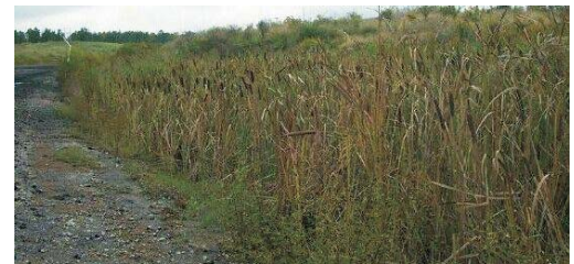
Roadside ditch bottom protected by vegetated Recyclex.
