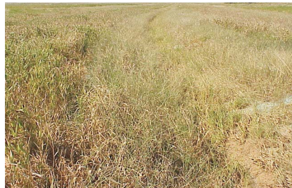
Drainage channel with fully established reinforced vegetation system.
